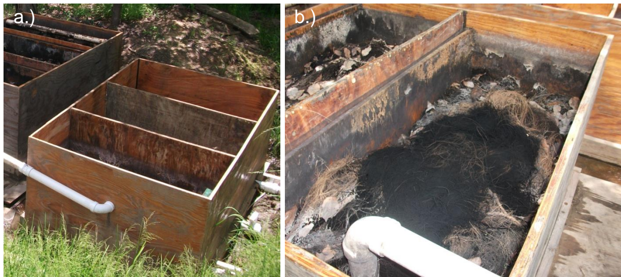
Fig. 2. Metal removal units. A metal removal unit at the passive coal mine drainage treatment site near Glasgow, PA.
